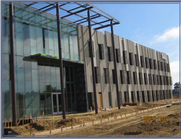
ECOB during final stages of construction
